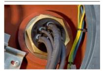
Indirect cable entry, very high safety level from type of protection increased safety sec and flameproof enclosure adc.
